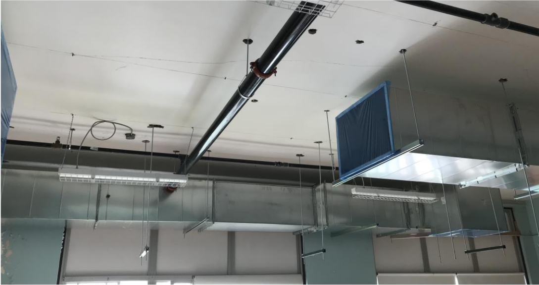
Duct and Sprinkler Pipe Install
