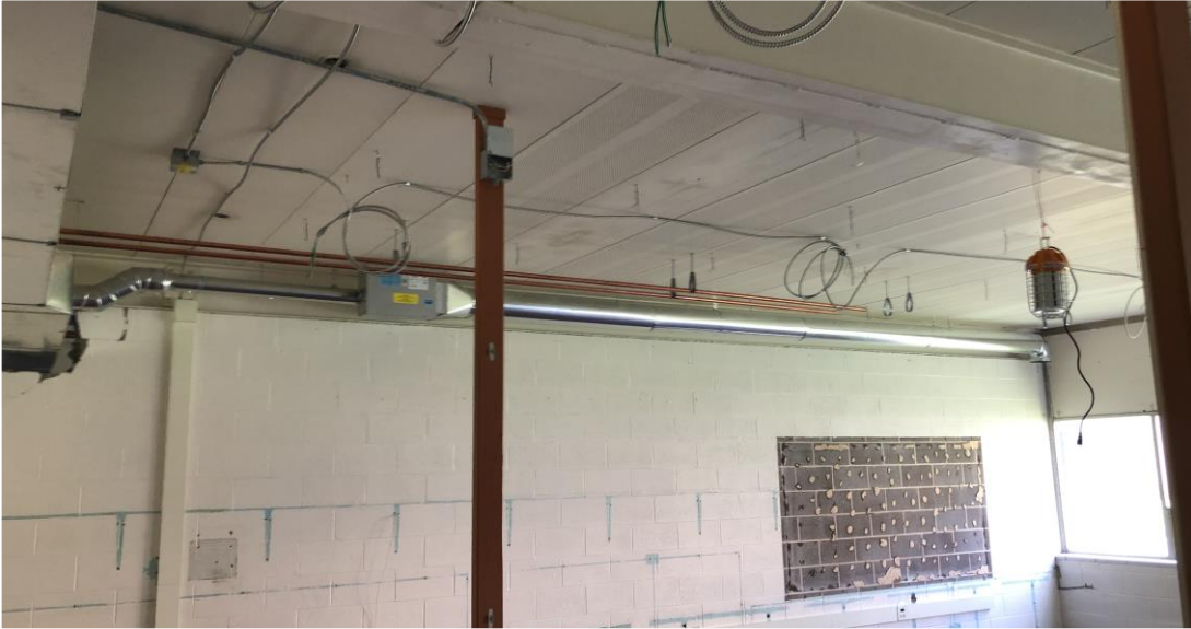
Duct and VAV Install
