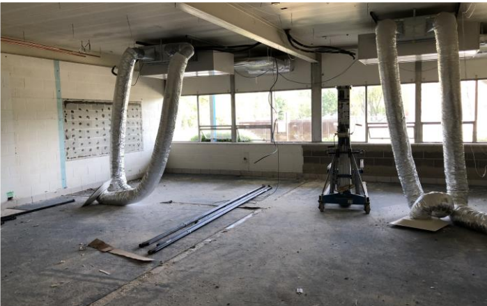
Duct and VAV Install
