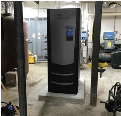
Boiler Placement
