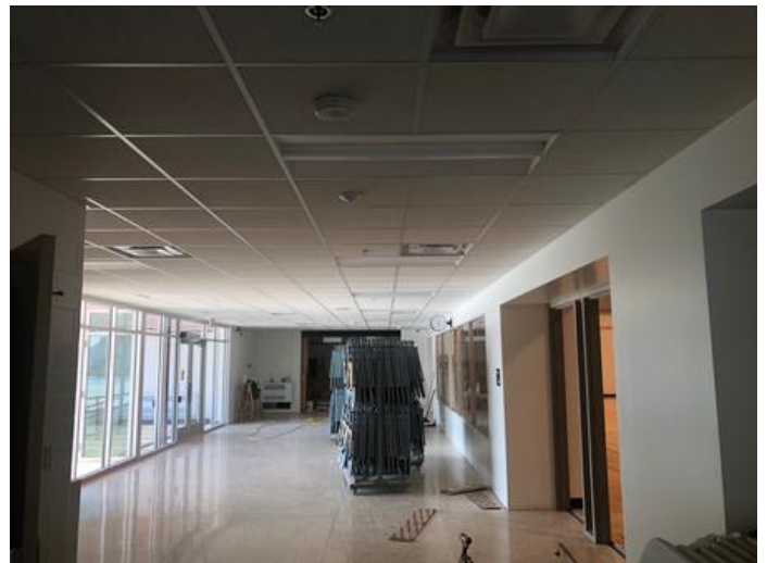
Ceiling Tile Install
