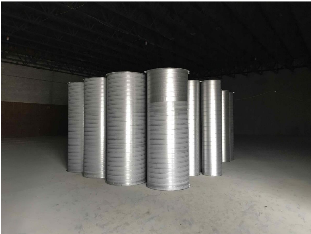
Gym Ductwork Delivery
