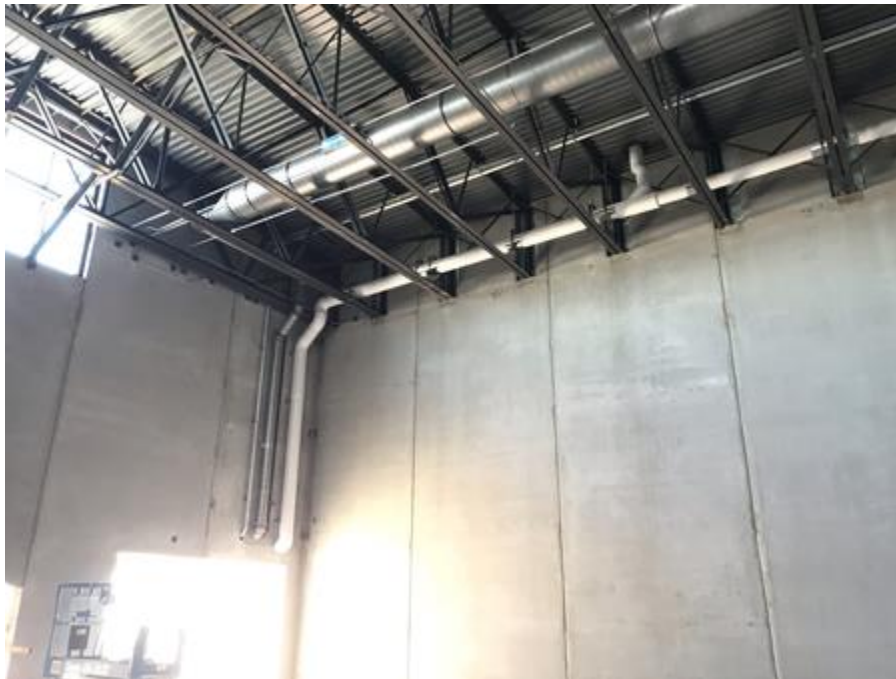
Gym Addition Progress
