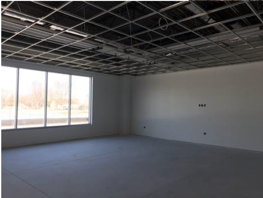
Classroom Ceiling Installation
