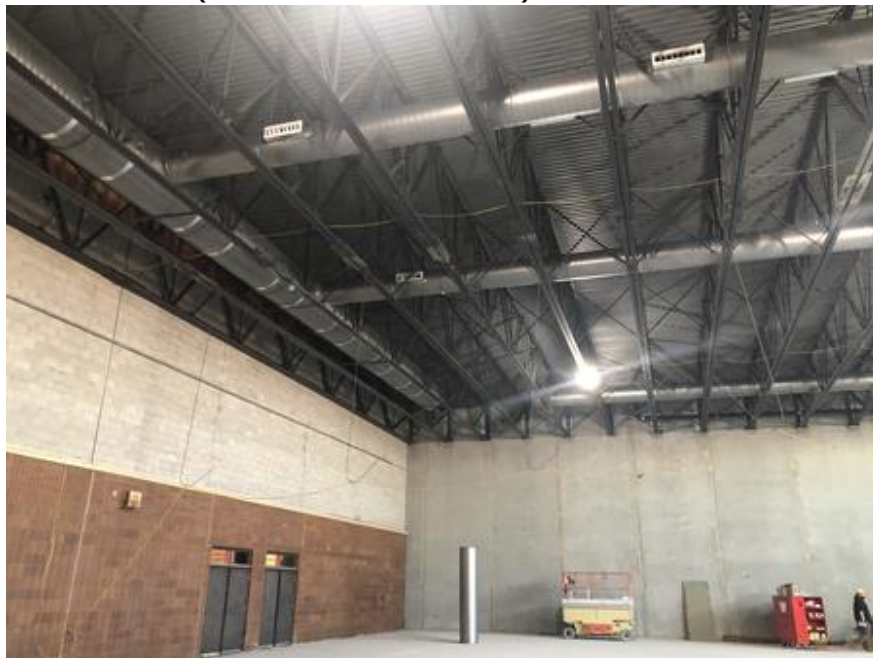
Ductwork Installation
