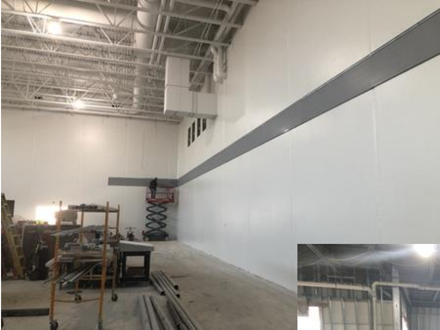
Finned Tube Radiation Install
